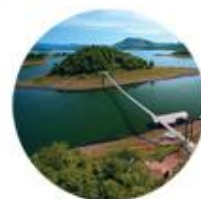
Kaengkrachan Dam (佛丕府)
